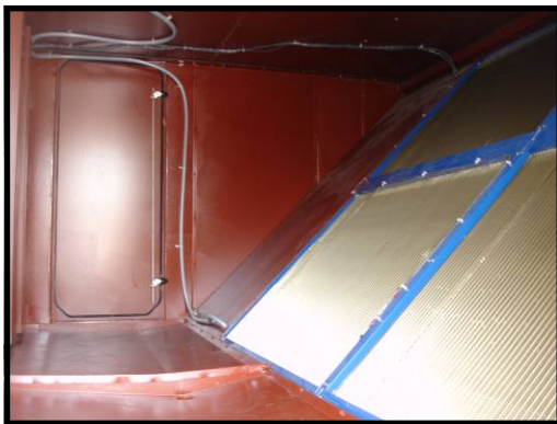
Heresite-Coated Cabinet Interior and Epoxy-Coated Exchanger
