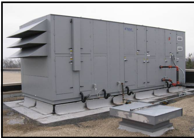
The Finished and Installed PXHS
