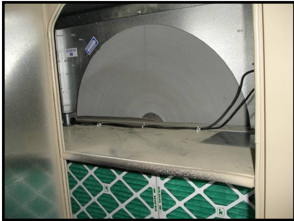
Heat Wheel and Filters
