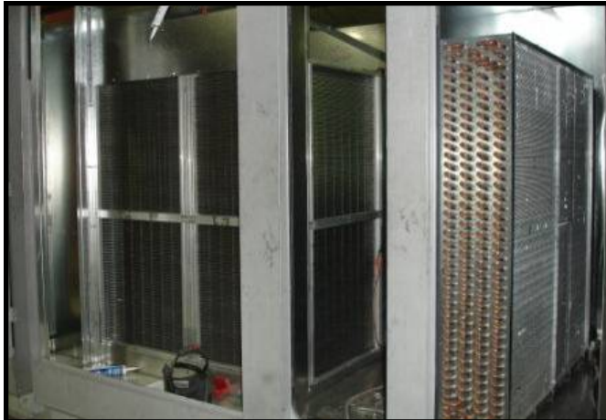
The heat exchanger (left) and cold water coil (right). The exchanger is flat, creating no turns within the unit.
