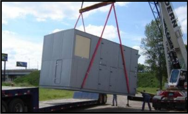
Unit being loaded onto a double-drop deck trailer for shipment.
