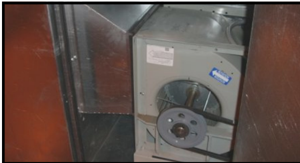
Blowers are forward curved, DWDI, class I and are arranged in a draw through configuration for quiet and efficient operation. Motors are high efficient, ODP, T-frame, 1750 rpm, 1.15 service factor and are mounted on adjustable bases with variable pitch sheaves. Motor and blower are mounted on common frames, isolated from unit case with RIS (spring optional) isolators, and have flexible duct connections.
