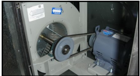
Blowers are forward curved, DWDI, class I and are arranged in a draw through configuration for quiet and efficient operation. Motors are high efficient, ODP, T-frame, 1750 rpm, 1.15 service factor and are mounted on adjustable bases with variable pitch sheaves. Motor and blower are mounted on common frames, isolated from unit case with RIS (spring optional) isolators, and have flexible duct connections.
