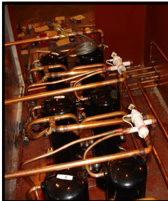
XeteX completely plumbed the refrigeration circuit and provided all wiring and controls.
