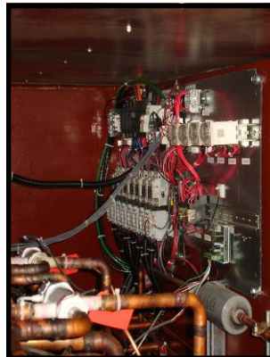
XeteX completely plumbed the refrigeration circuit and provided all wiring and controls.
