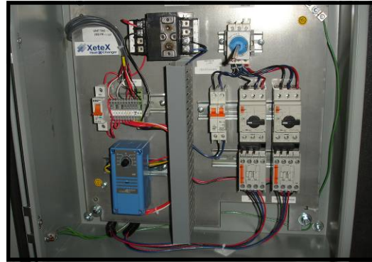
An XeteX Control Panel with Analog Controls (the blue stat appears on the lower left side).
